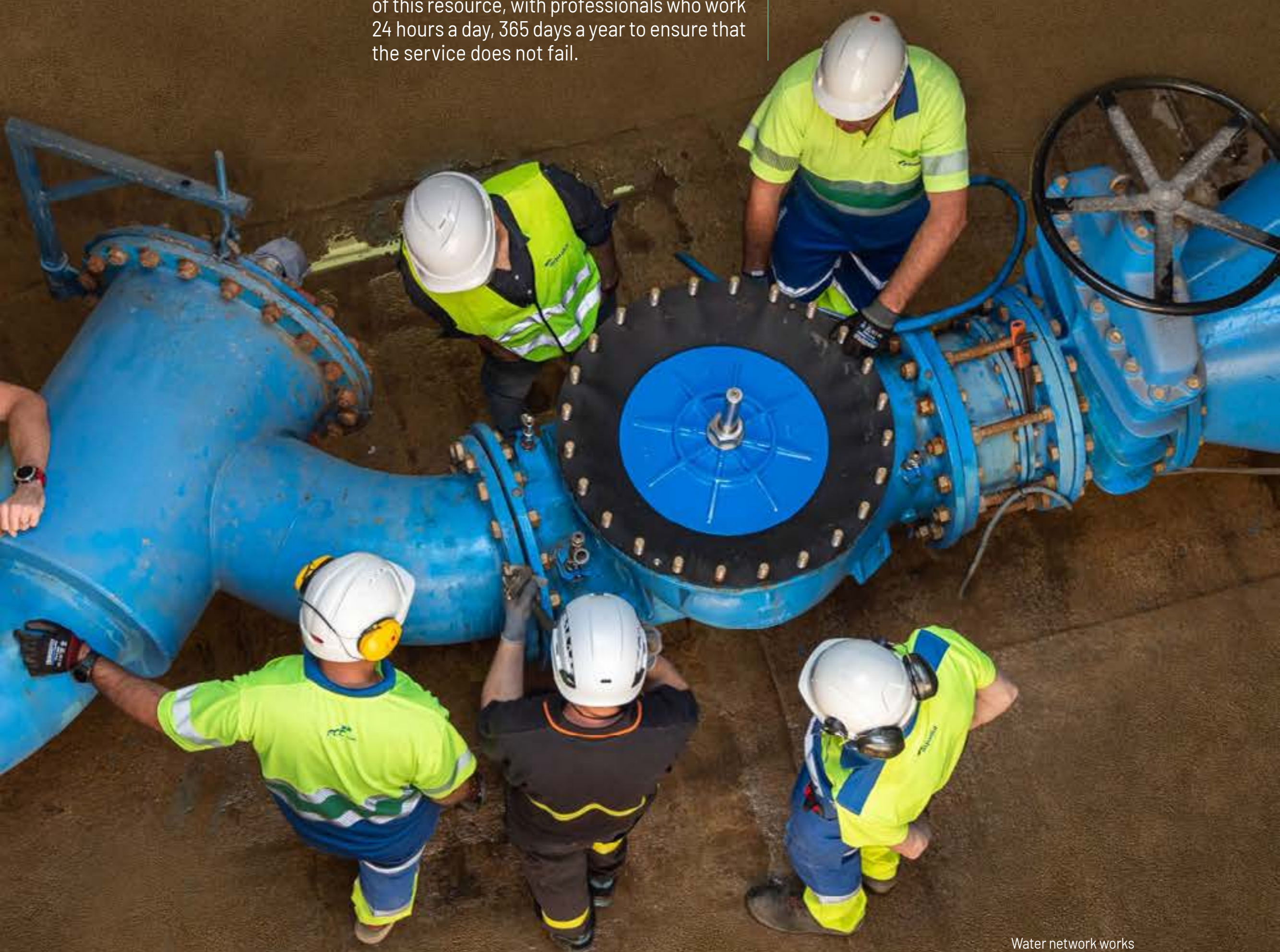
Water network works
